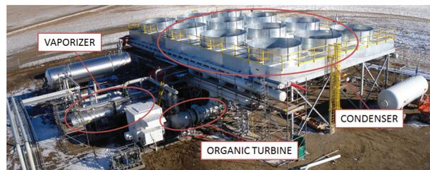
Fig. 3. ORC utilization unit 6MW power working at gas compressor station in Loreburn (Canada) [11]
